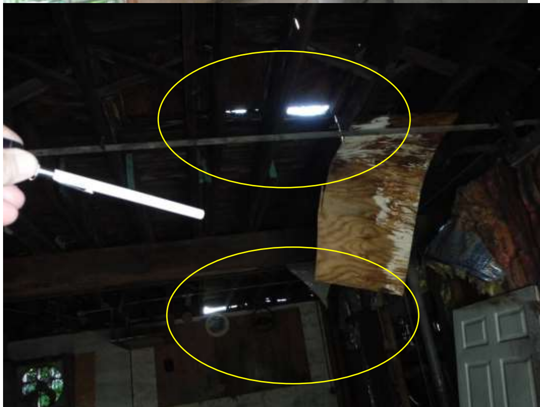
Figure 6 Roof deteriorated; daylight, leaks, rot, damage everywhere. Recommend a building contractor evaluate advise on roof structure & roof removal/replacement.
